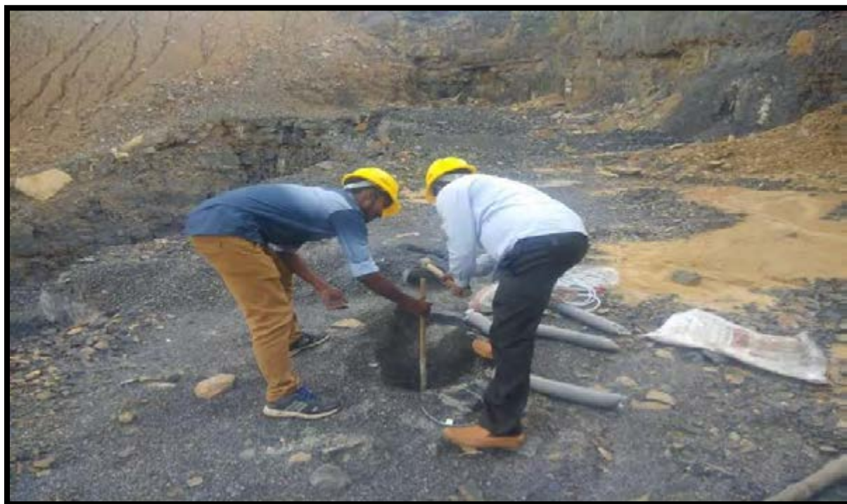
Fig.11(c): Stemming using Crushed Aggregate for blasting at Tamoria Mine
