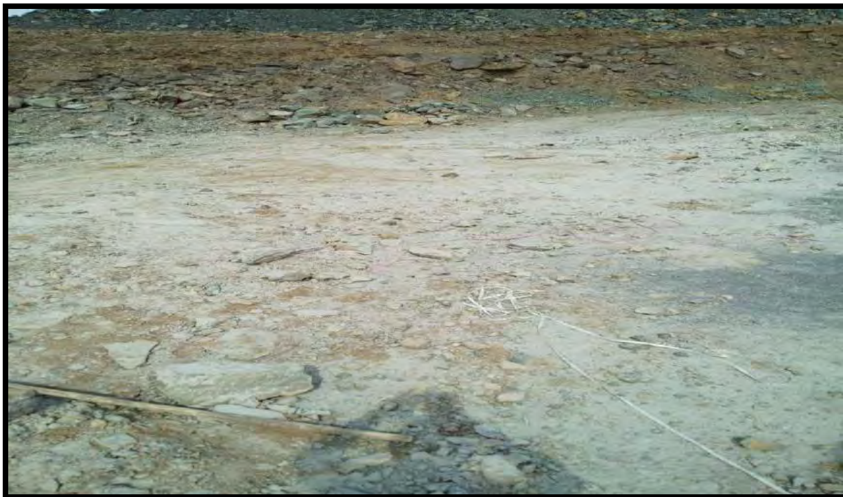
Fig.11(b): Bench Preparation for blasting at Tamoria Mine
