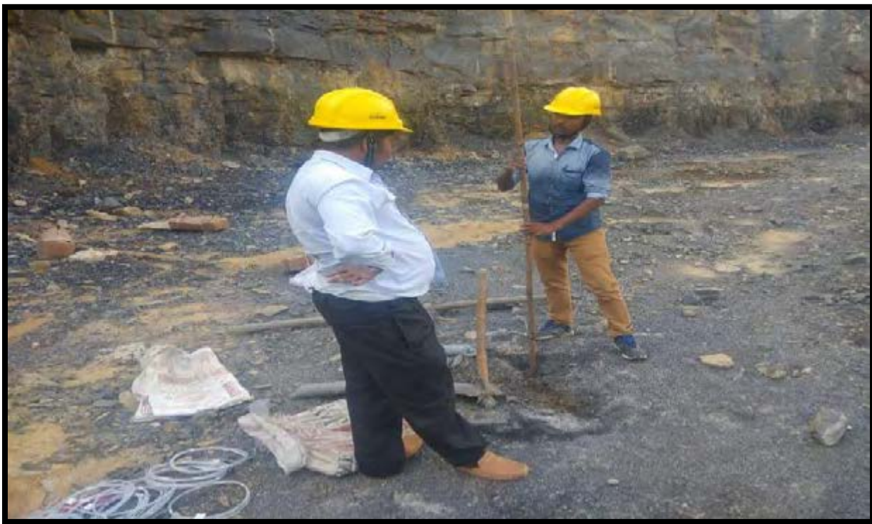
Fig.10: Stemming with Crushed Aggregate Material
