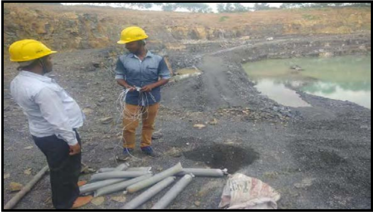
Fig.11(d): Explosive Charging for blasting at Tamoria Mine
