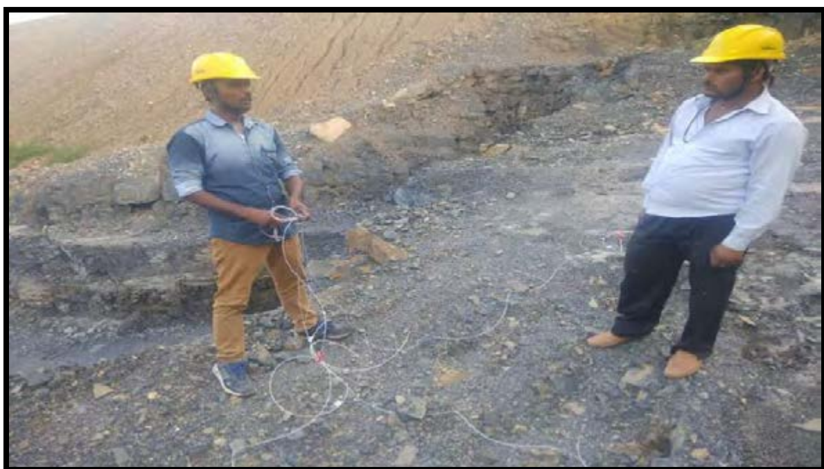
Fig.11(a): Surface Connections Using Nonel
