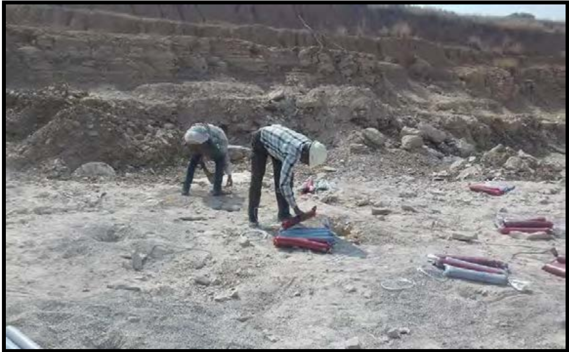
Fig.8: Charging of Blast Hole using Emulsion Cartridges (Shankh Prime)
