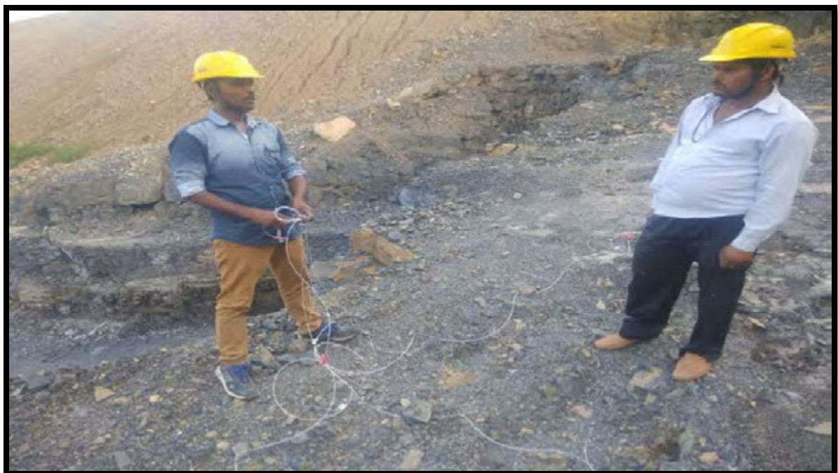
Fig.11(a): Surface Connections Using Nonel
