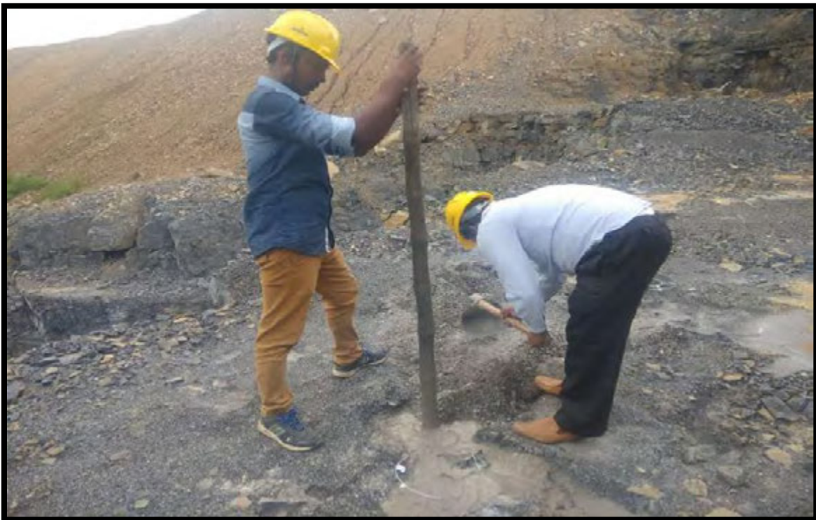
Fig.9: Water in Blast Hole and Loading of Stemming Material
