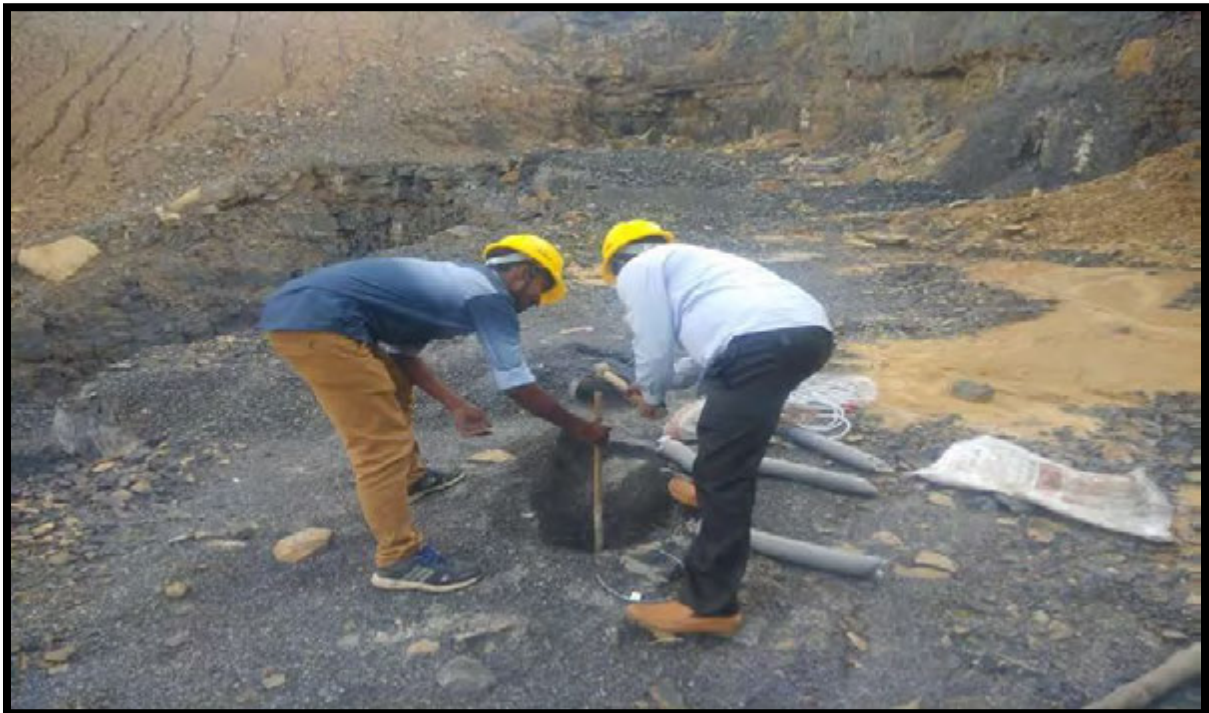
Fig.11(c): Stemming using Crushed Aggregate for blasting at Tamoria Mine
